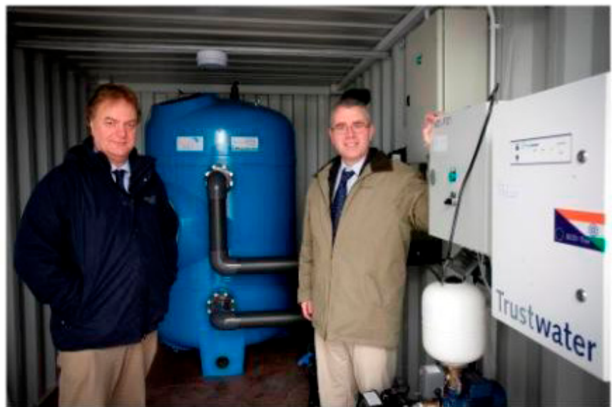
Cutting-edge integrated European systems for water disinfection (Trustwater ECO-Trio) and filtration (Dryden Aqua AFM, background) for installation at a rural community pilot site in West Bengal, India (Credit: Hume Brophy)
